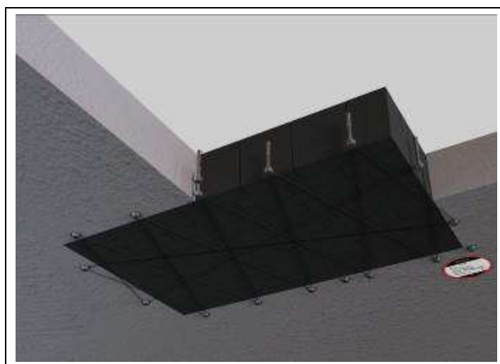
Figure A.4: Example of reinforcement net for a blank penetration seal in floors.
